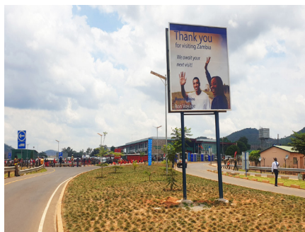
Figure 2: One-stop border infrastructure and customs turn-style checkpoint facilities in Zambia, Africa.
